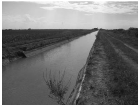
Figure 5. Ground-level photograph of a concrete canal section in the Delta Lake Irrigation District (Case 1)
