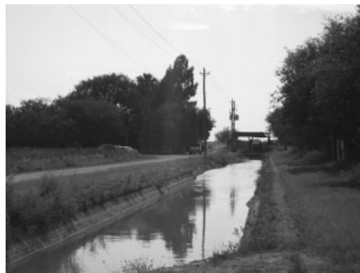
Figure 7. Ground-level photograph of a concrete canal section in the Delta Lake Irrigation District (Case 2)
