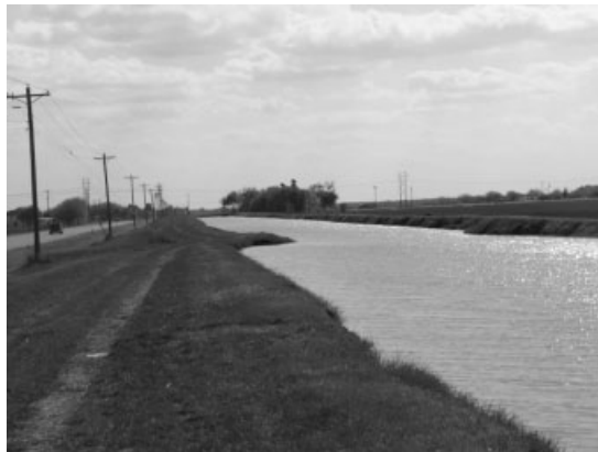
Figure 9. Ground-level photograph of an earth canal section in Harlingen Irrigation District 2 (Case 3)
